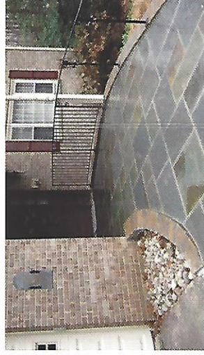
Flagstone Ramp entrance zero threshold. No steps
