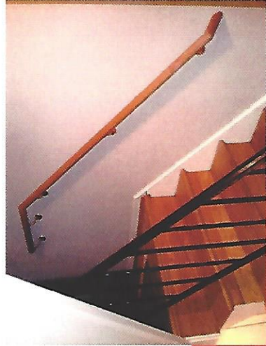
Handrail on both sides of the stairs
